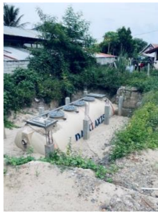
Backfilling
