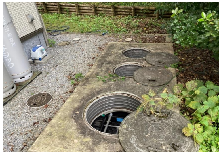
Johkasou System operated by Nasu Create (in Japan)
