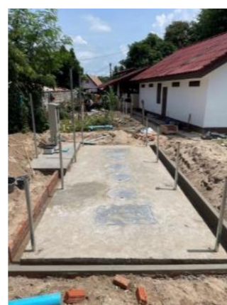
Slab casting
